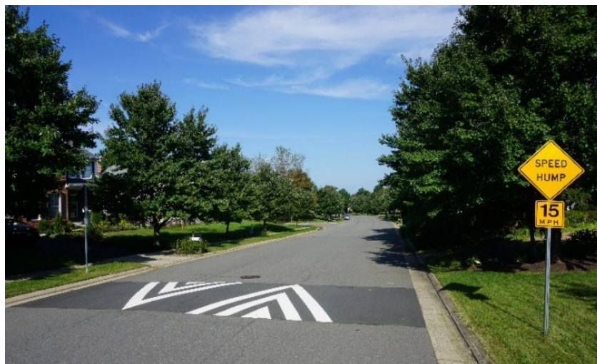
Figure 6. Speed Hump on Farmingdale Drive in Ashburn Farm Community
