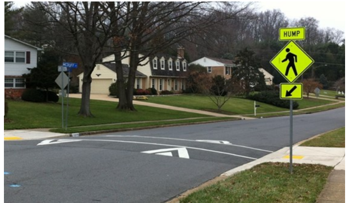
Typical Raised Crosswalk Application Source: VDOT Traffic Calming Guide for Neighborhood Streets
