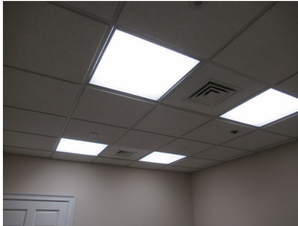
Acoustical ceiling tile and grid system
