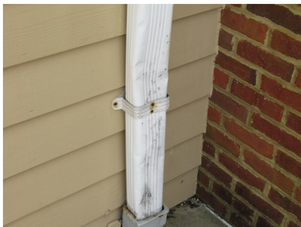
Downspout fastener rust and damage
