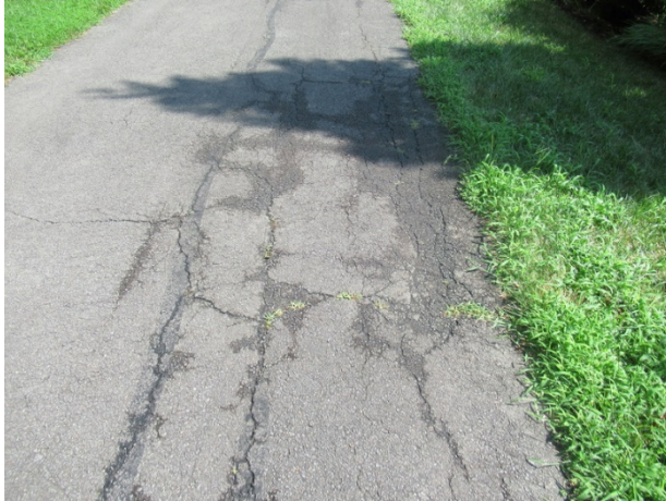
Asphalt pavement walking path cracks and deterioration
