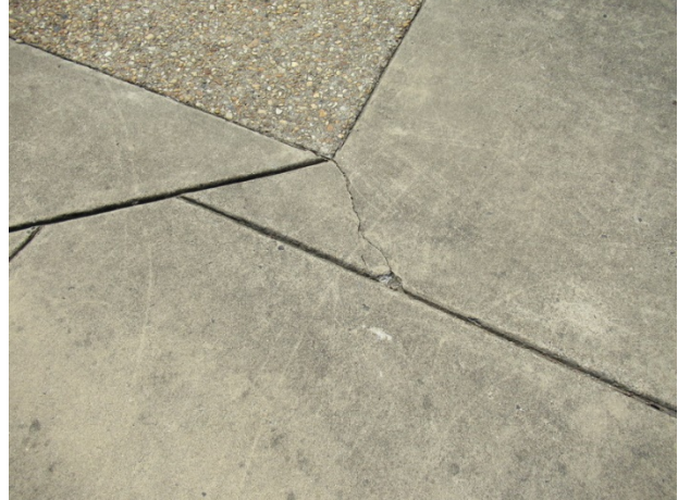
Concrete sidewalk crack
