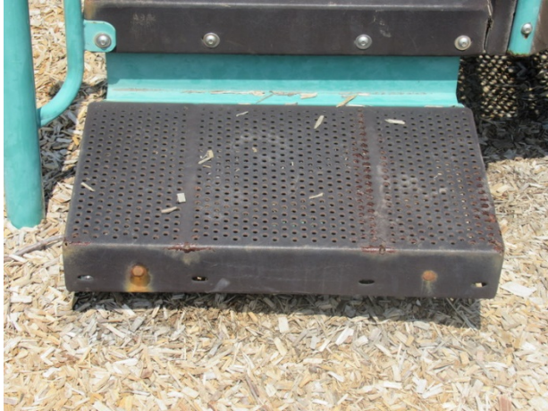
Finish deterioration and rust
