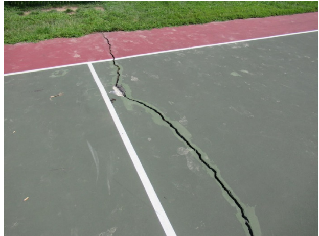
Basketball court crack and deterioration
