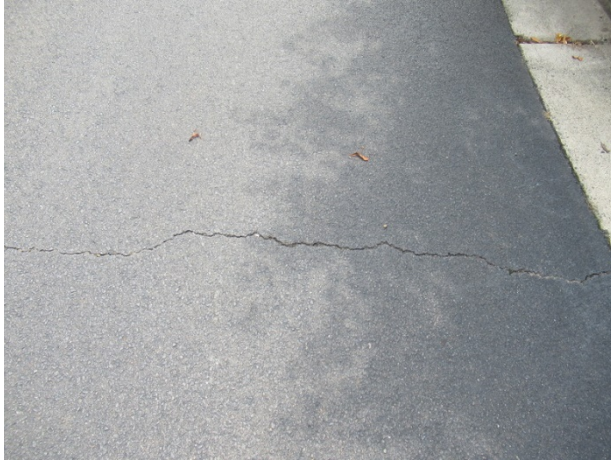
Asphalt pavement crack
