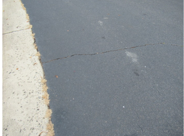
Asphalt pavement crack
