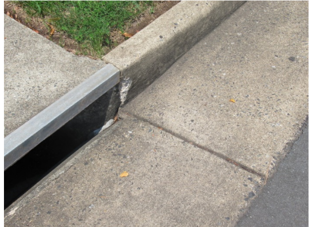
Concrete curb spall
