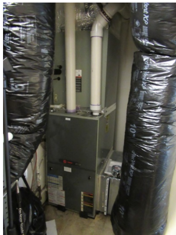
Interior air handling unit
