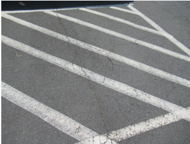
Asphalt pavement cracks
