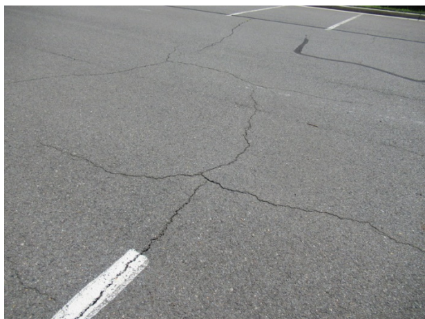
Asphalt pavement cracks
