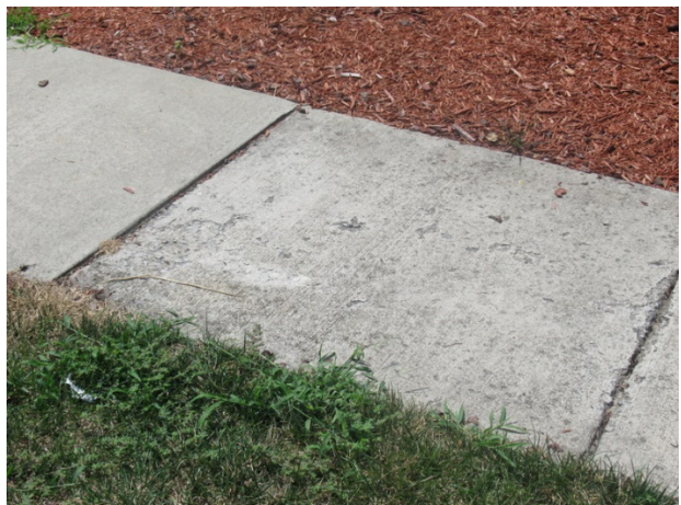
Concrete sidewalk scaling
