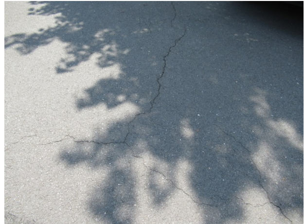
Asphalt pavement cracks
