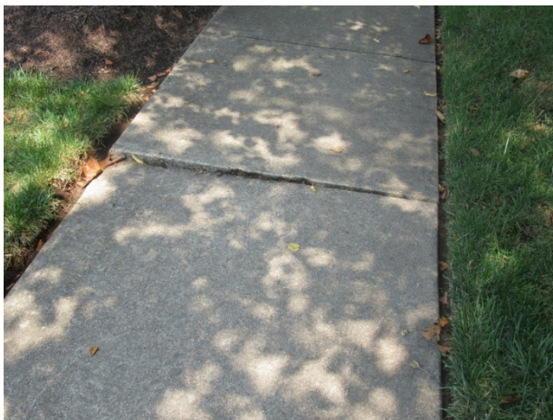
Concrete sidewalk trip hazard
