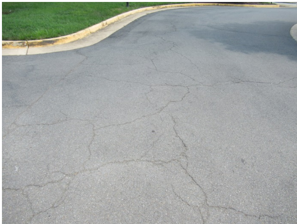
Asphalt pavement cracks and deterioration
