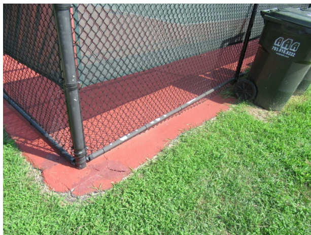
Finish deterioration
