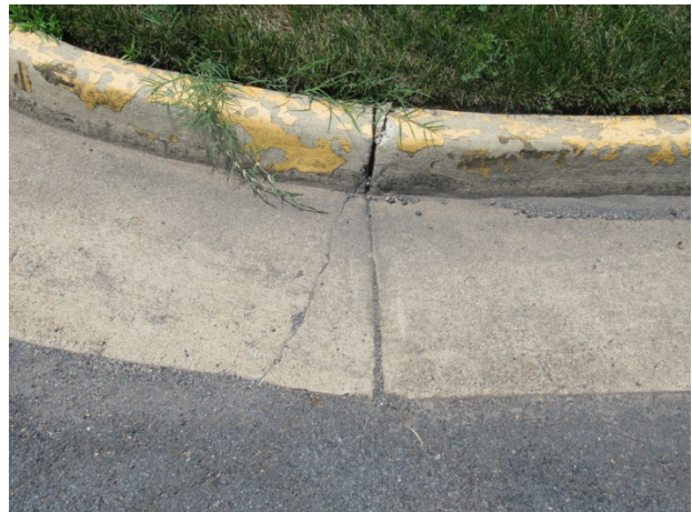
Concrete curb and gutter crack
