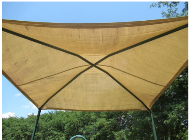
Shade structure fabric deterioration
