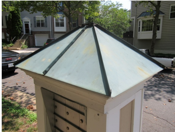
Metal roof finish deterioration
