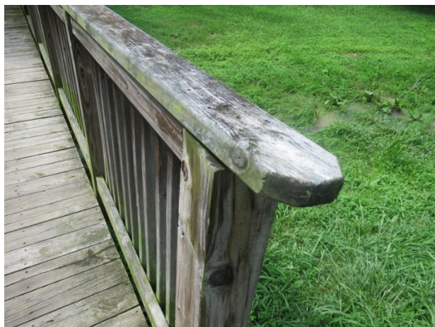
Organic growth and railing deterioration
