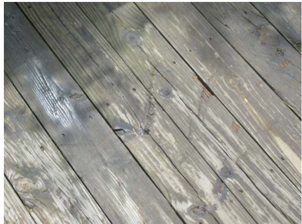
Deck board deterioration
