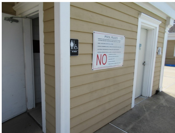
Siding finish deterioration
