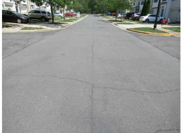
Asphalt pavement overview – Note: cracks
