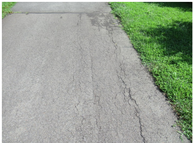
Asphalt pavement walking path cracks and deterioration
