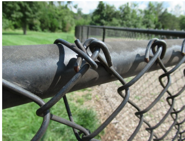
Chain link fence finish deterioration
