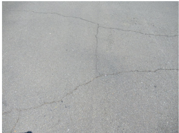
Asphalt pavement cracks
