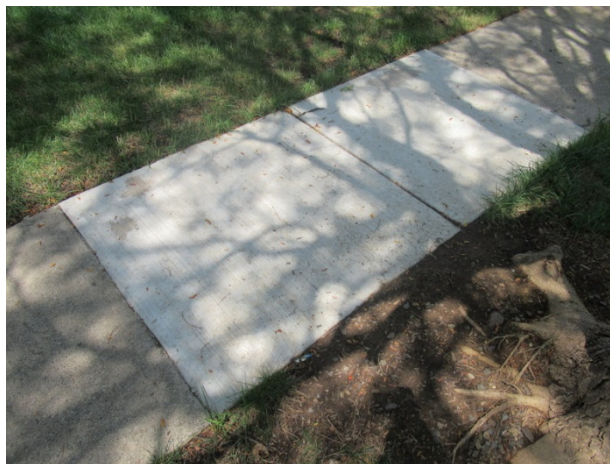
Replaced section of concrete sidewalk
