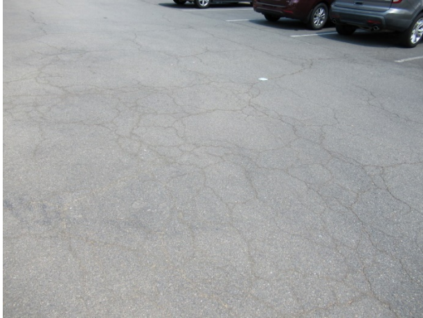
Asphalt pavement cracks and deterioration
