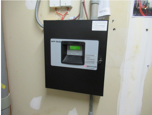
Life safety system control panel
