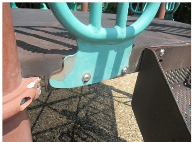
Finish deterioration and rust
