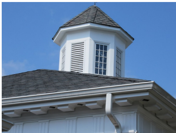
Asphalt shingle roof assembly
