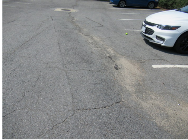
Asphalt pavement cracks
