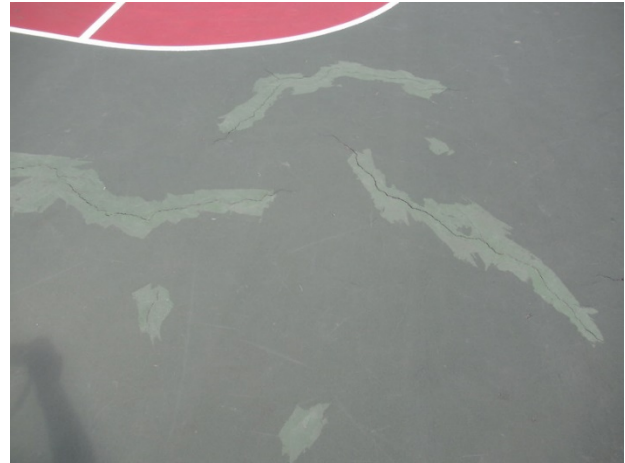
Repairs, cracks and color coat deterioration
