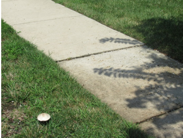
Concrete sidewalk trip hazard
