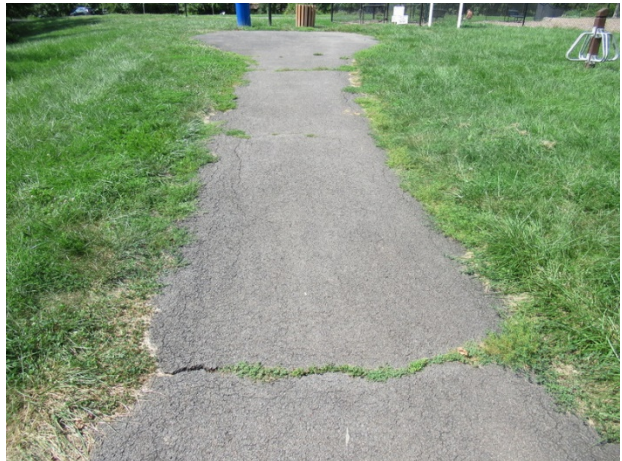
Asphalt pavement walking path crack
