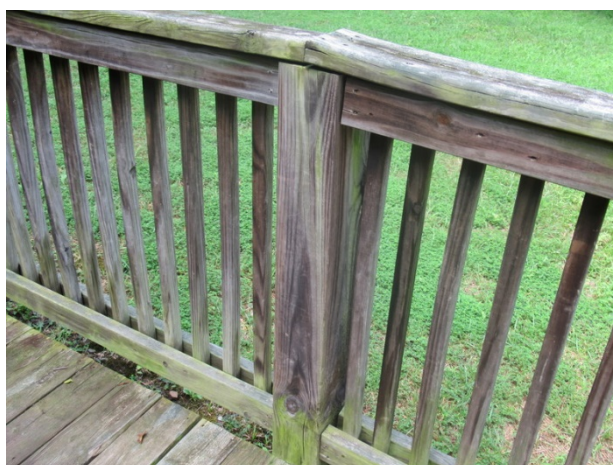
Organic growth and railing deterioration
