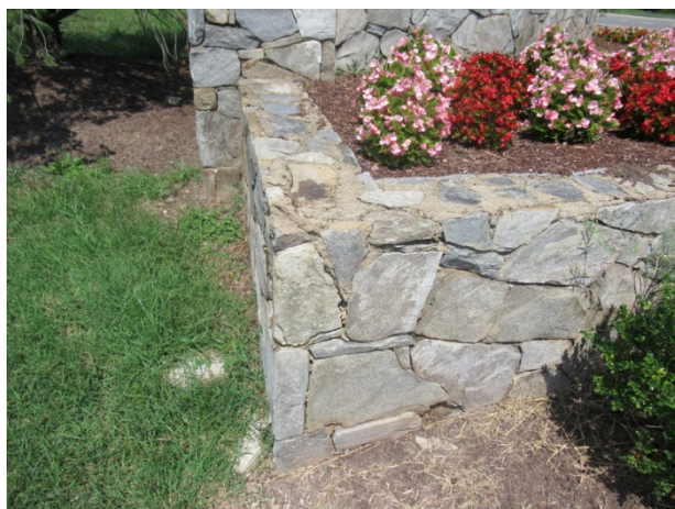
Mortar deterioration
