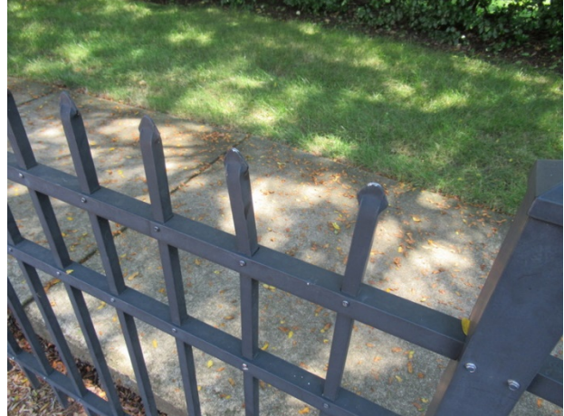
Aluminum fence damage and finish deterioration
