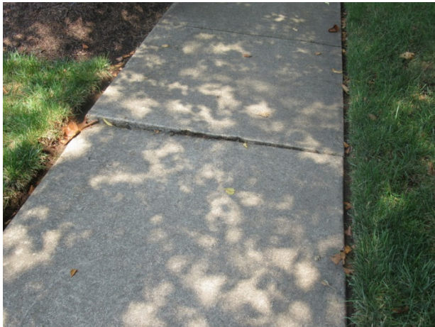
Concrete sidewalk trip hazard
