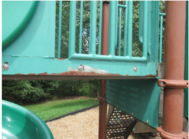
Finish deterioration and rust
