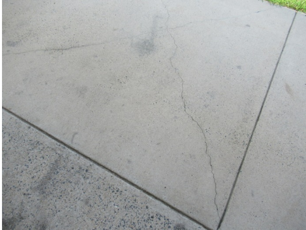
Concrete sidewalk cracks
