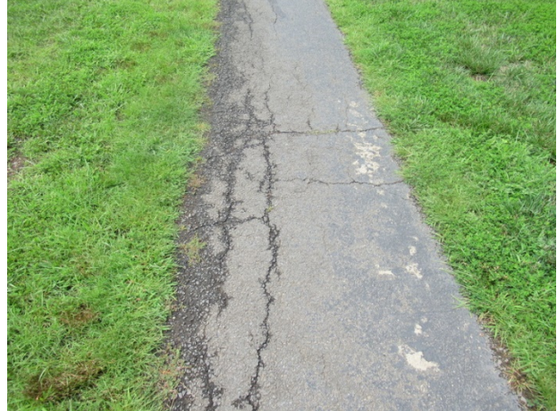
Asphalt pavement walking path cracks and deterioration
