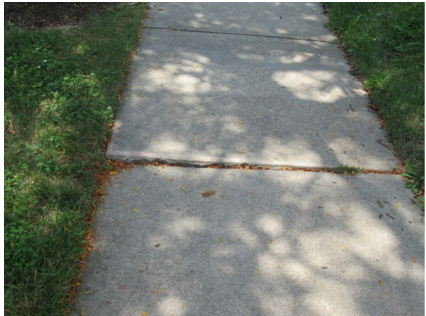
Concrete sidewalk trip hazard
