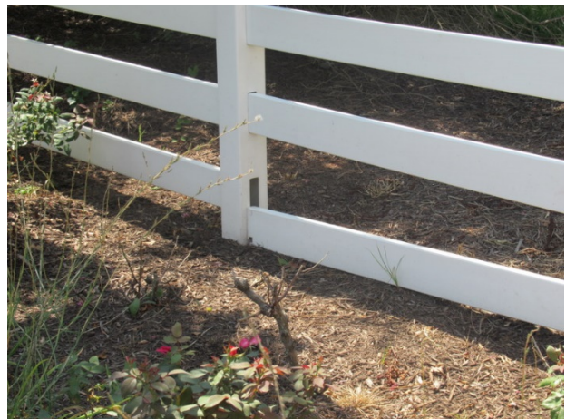
Rail displacement
