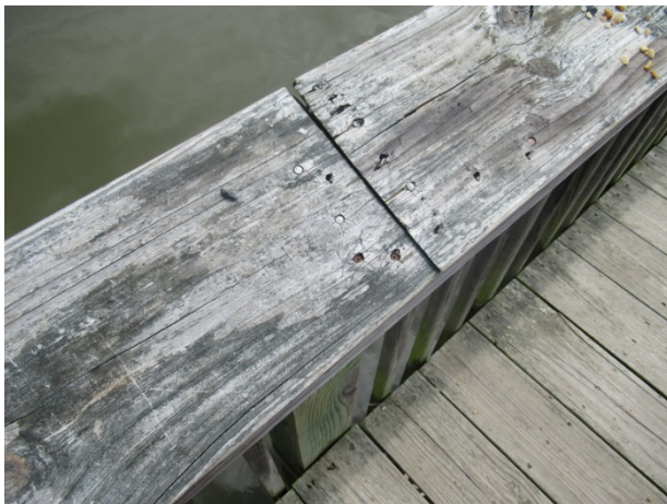
Finish pier railing deterioration and fastener rust
