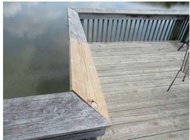
Replaced section of railing
