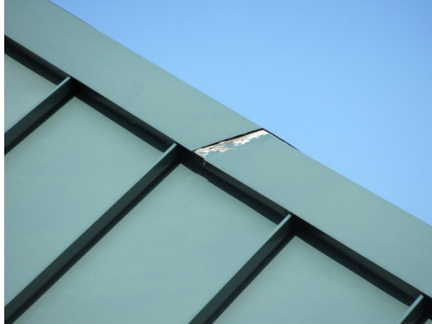
Metal roof finish deterioration
