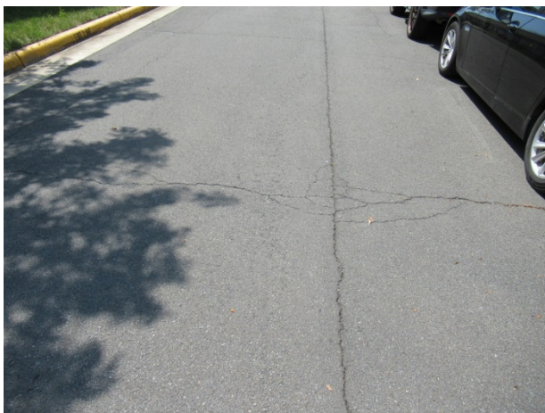
Asphalt pavement cracks
