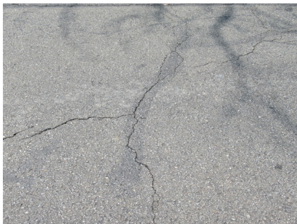
Asphalt pavement cracks
