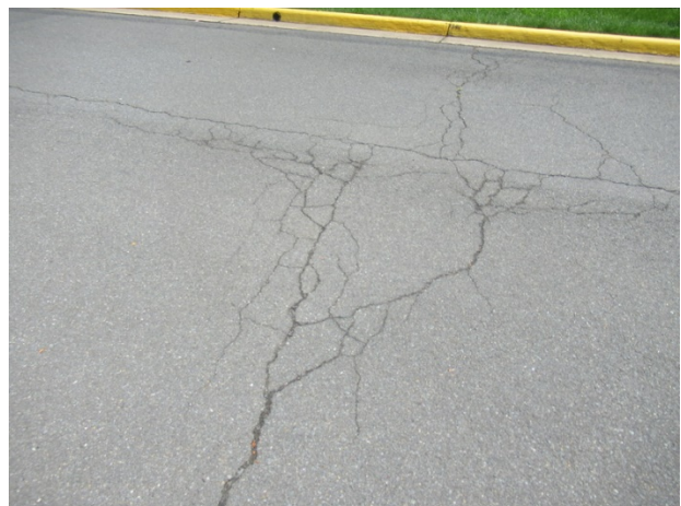
Asphalt pavement cracks and deterioration
