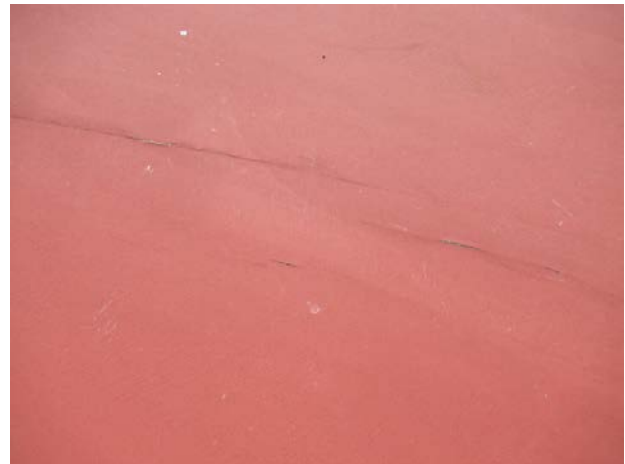
Murrey Park tennis court color coat deterioration and cracks
