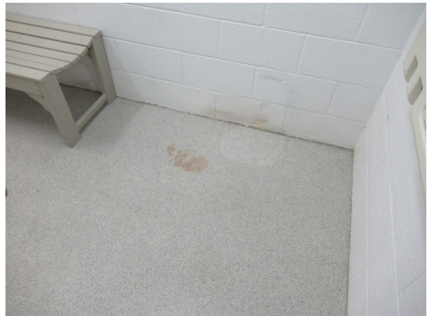
Epoxy floor deterioration
