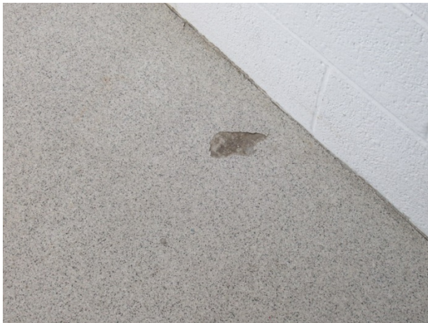
Epoxy floor deterioration
