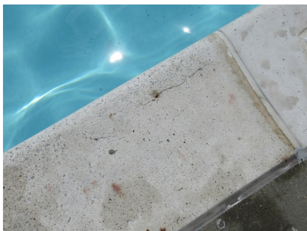
Main pool coping cracks
