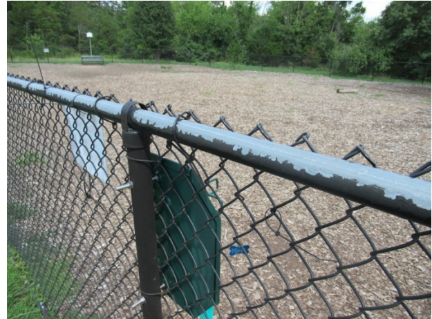
Chain link fence finish deterioration
