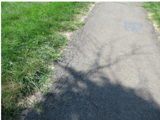
Asphalt pavement walking path cracks and deterioration
