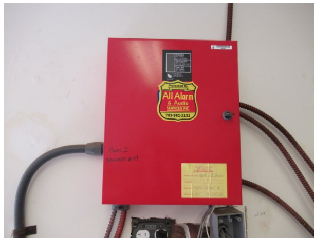
Life safety system control panel
