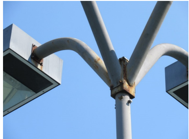
Finish deterioration and rust at Town Hall tennis court light poles and fixtures
