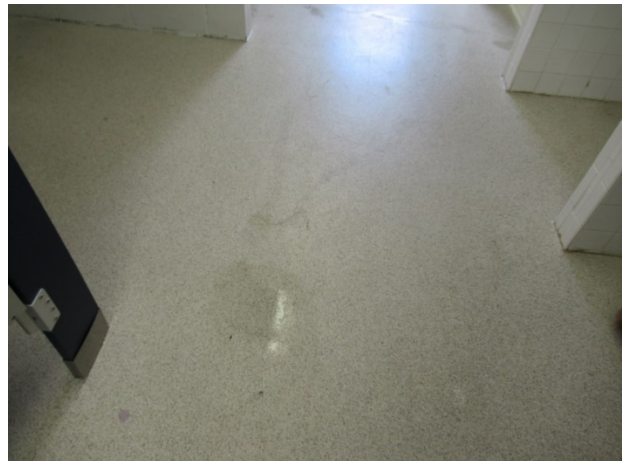
Epoxy floor coating deterioration
