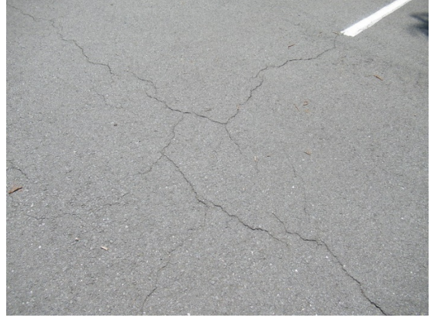
Asphalt pavement cracks
