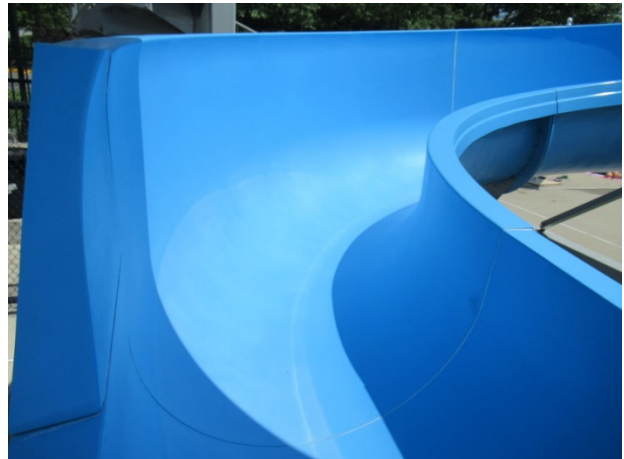
Finish deterioration at main pool slide
