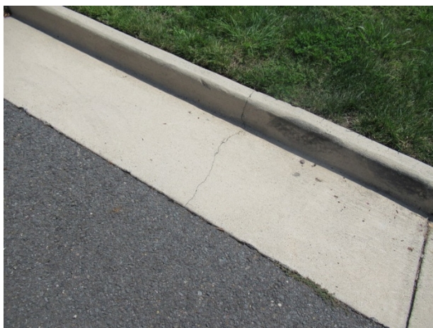
Concrete curb and gutter crack
