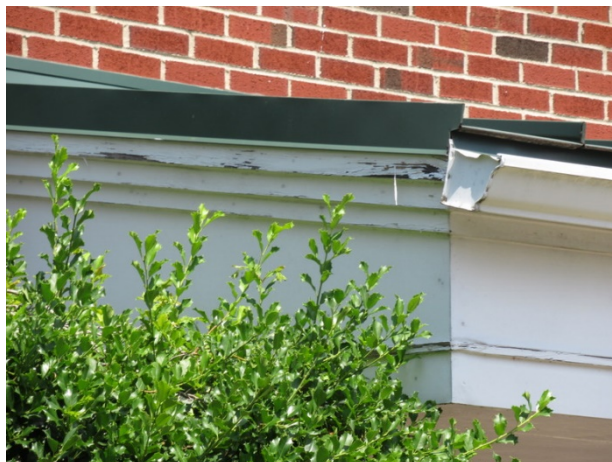
Trim deterioration
