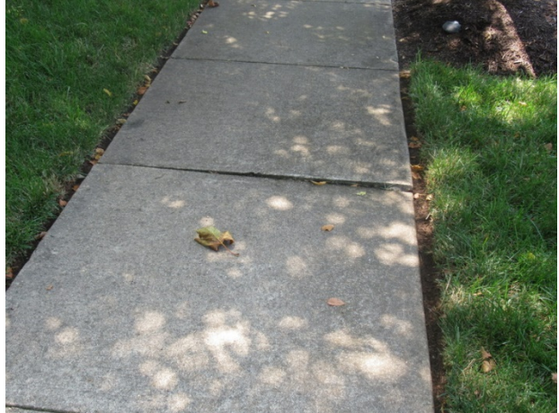
Concrete sidewalk trip hazard
