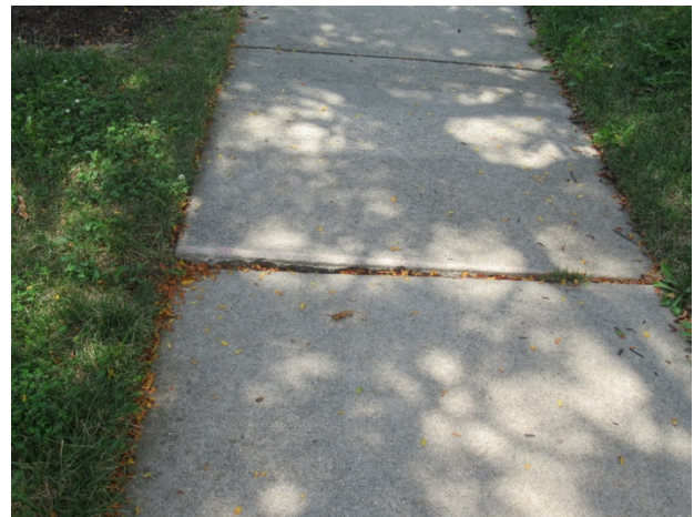
Concrete sidewalk trip hazard
