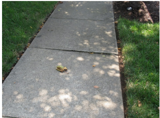
Concrete sidewalk trip hazard
