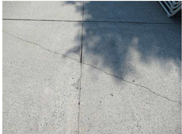
Concrete deck crack
