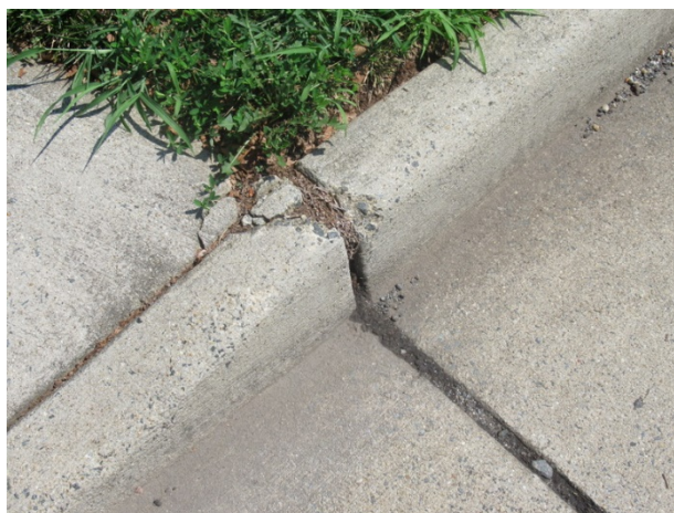
Concrete curb spall
