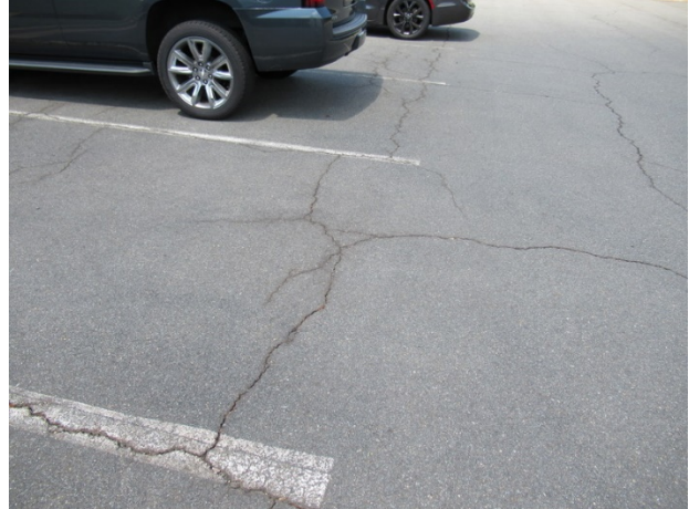
Asphalt pavement cracks
