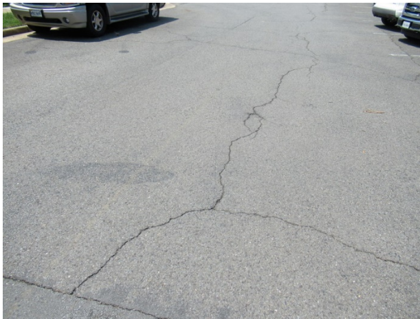
Asphalt pavement cracks
