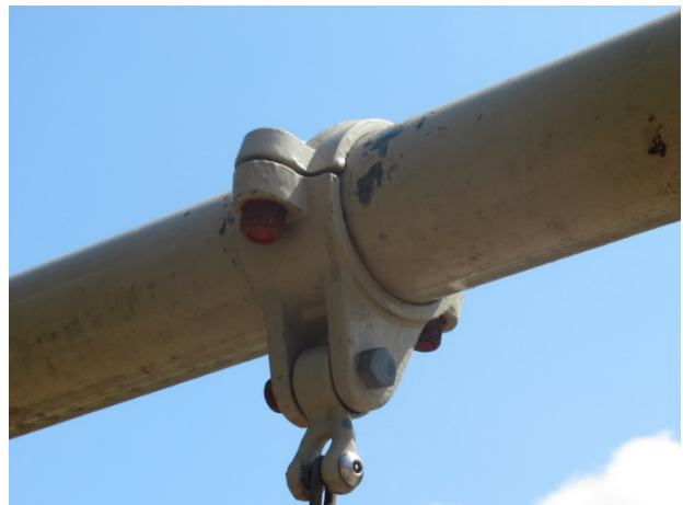
Finish deterioration and rust
