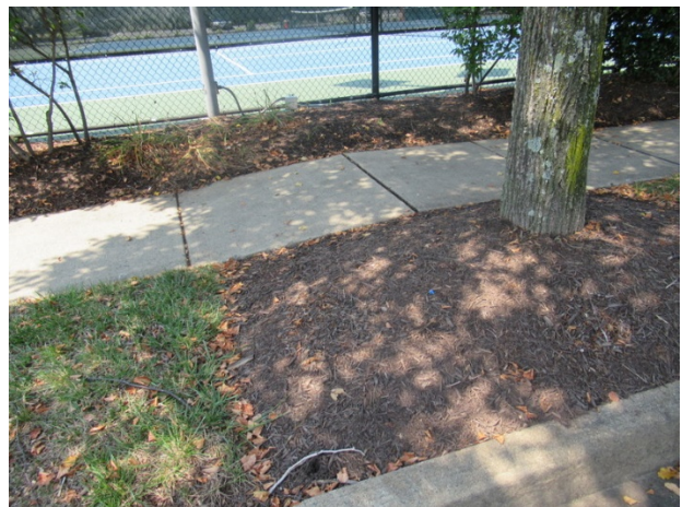
Concrete sidewalk heave
