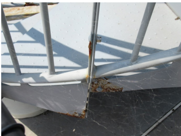
Main pool slide staircase rust
