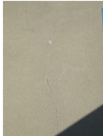
Concrete deck crack
