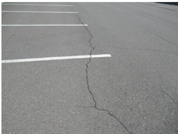
Asphalt pavement cracks
