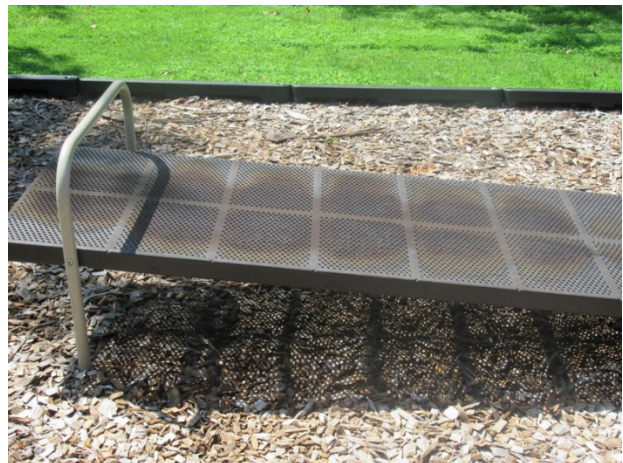
Finish deterioration
