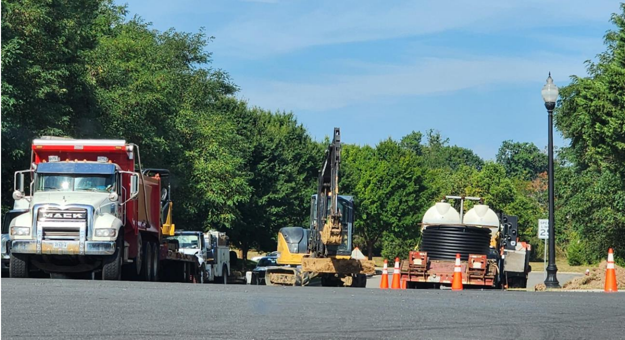
8/30/23: Photo - showing infrastructure installations underway.
