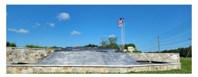
**3/15/2024:** We were notified that the waterproofing liner installation is complete. We are waiting for temperatures to remain above freezing to turn on our irrigation system (our water source for this project) to complete the water test to ensure the fountain is holding.
