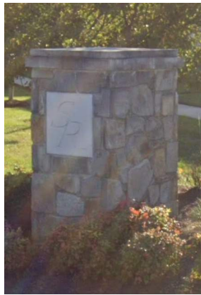
SOUTH RIDING COLUMNS REFERENCE IMAGERY
