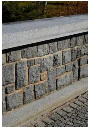
SEATWALLS STACKED STONE & CONCRETE CAP
