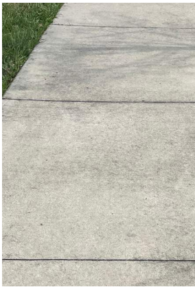
CONCRETE PATH STANDARD BROOM FINISH
